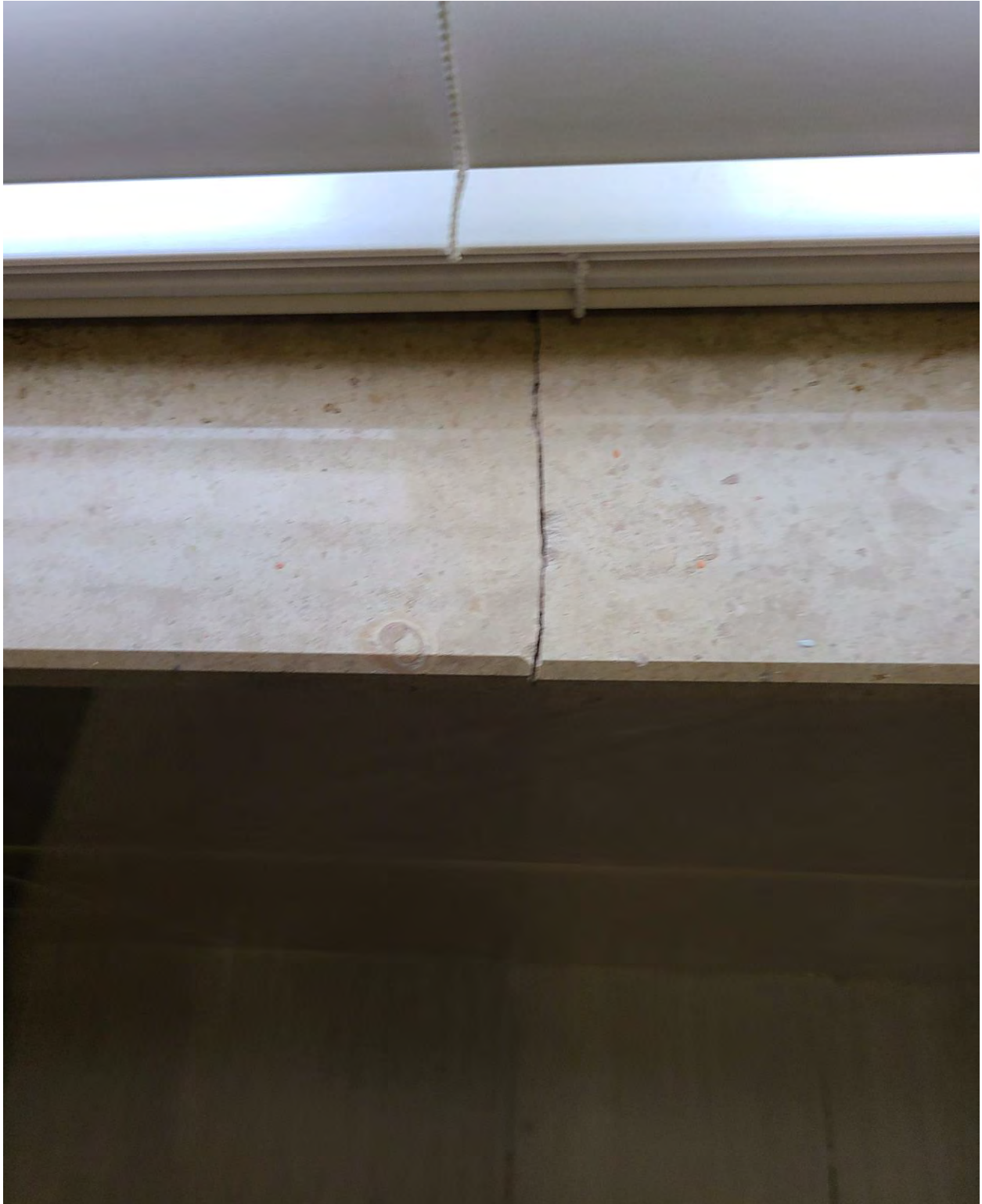
Broken Window Sill in Fitness Center Bathroom (Before):
